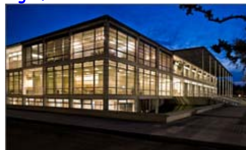
The Lavin-Bernick Center for University Life in New Orleans, Louisiana, is oriented to take advantage of prevailing breezes. Walls cooled with chilled water and air-cooled metal ceilings help to keep the building comfortable during hot summer days.
